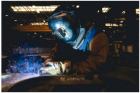
Albert Nelson structural welds on an aircraft carrier Enterprise unit. (Ashley Cowan/ Newport News Shipbuilding)
